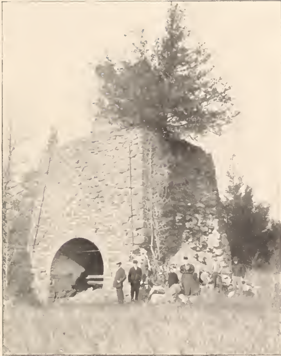
AETNA FURNACE, TUCKAHOE RIVER
